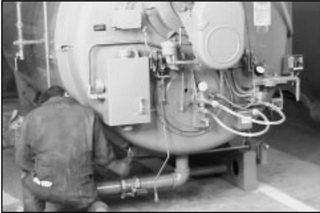
**Figure 8-35: Close and Tighten Front Head**
