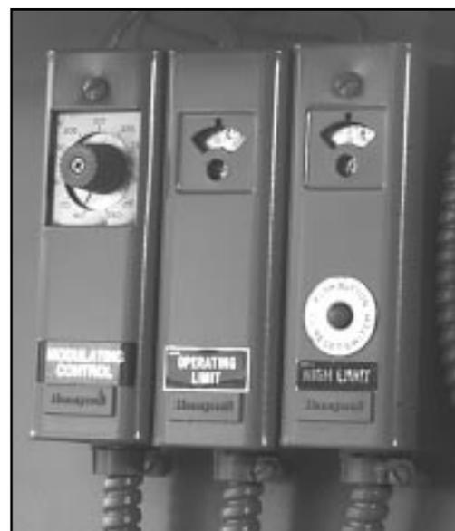
Figure: 6-5 Hot Water Controls
