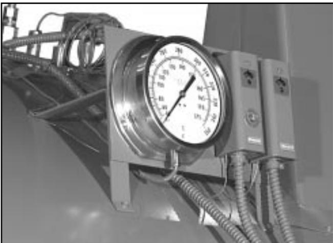
Figure: 1-11 Water Temperature Gauge
