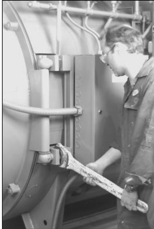
**Figure 8-36: Tighten Hinge Bolts**
