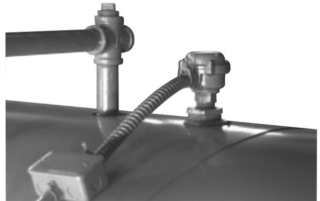
**Figure: 1-14 Auxiliary Low-Water Cutoff**
