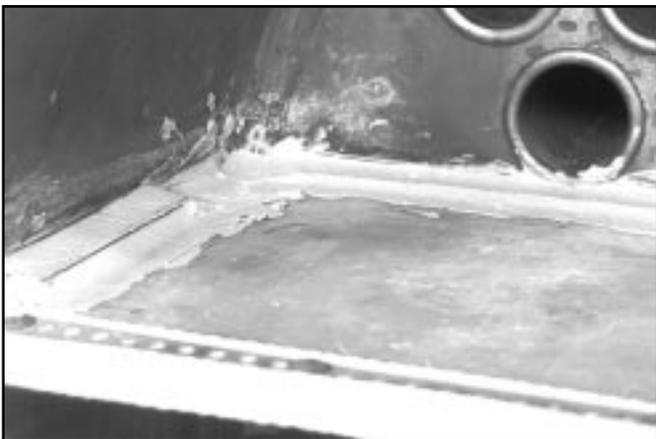
**Figure 8-28: High Temperature Cement on Baffle Weld Area**
