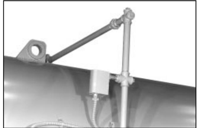
**Figure: 1-13 Low Water Cutoff (LWCO Hot Water)**
