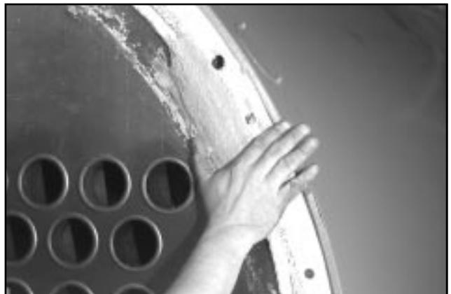
**Figure 8-30: Apply Pulp Over Rope and Tadpole Gasket**
