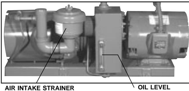
Figure: 5-7 Atomizing Air Compressor CB-LE (CB Option)
