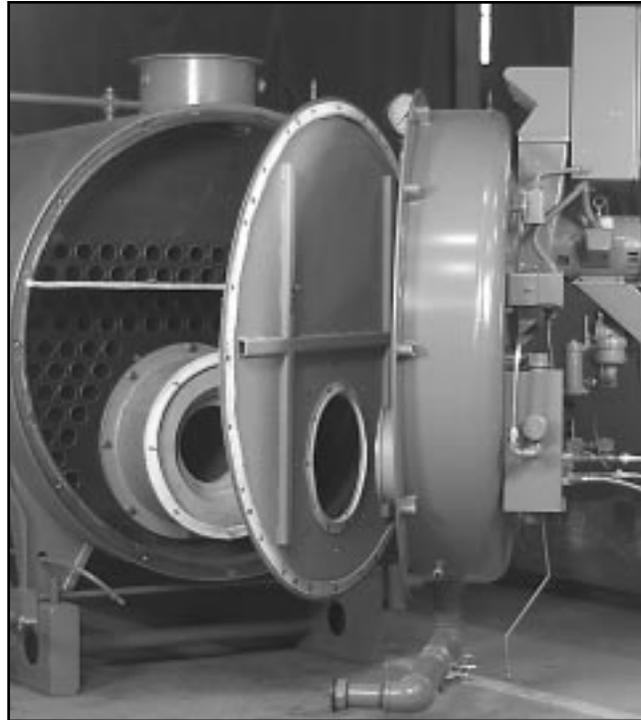
Figure 8-24: Open Front Head and Inner Door
