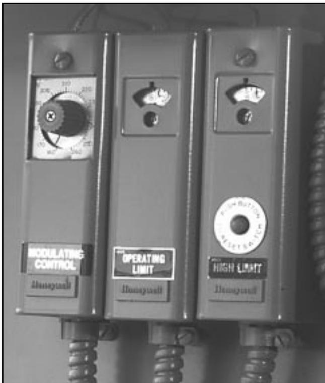
**Figure: 1-12 Hot Water Controls**
