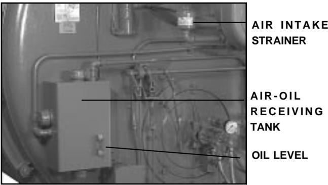
Figure: 5-5 Primary Air Strainer and Receiving Tank
