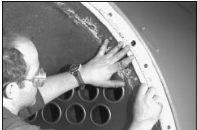
**Figure 8-29: Rope Gasket Glued against Tadpole Gasket**
